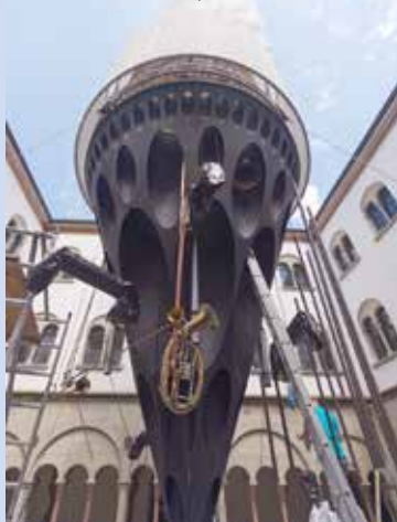
Rohrwerk, Grossmünster. Photo: Marc Delachaux, SAVE-EPFL
